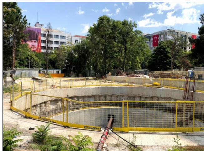
Figure 4.16. Subway construction at Zafer Park. Photograph taken by author.
