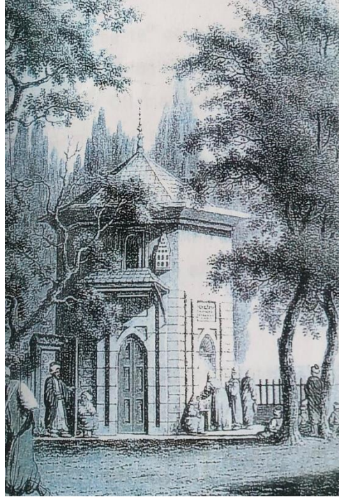
Figure 2.3. Water distribution station at Istanbul. (Source: Uludağ, 1998: 67)
